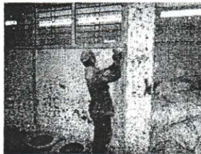
a) Extracting of wall
